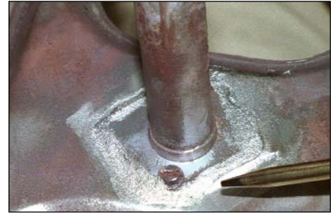
Pyro-Putty® 653 seals corroded burner manifold.
