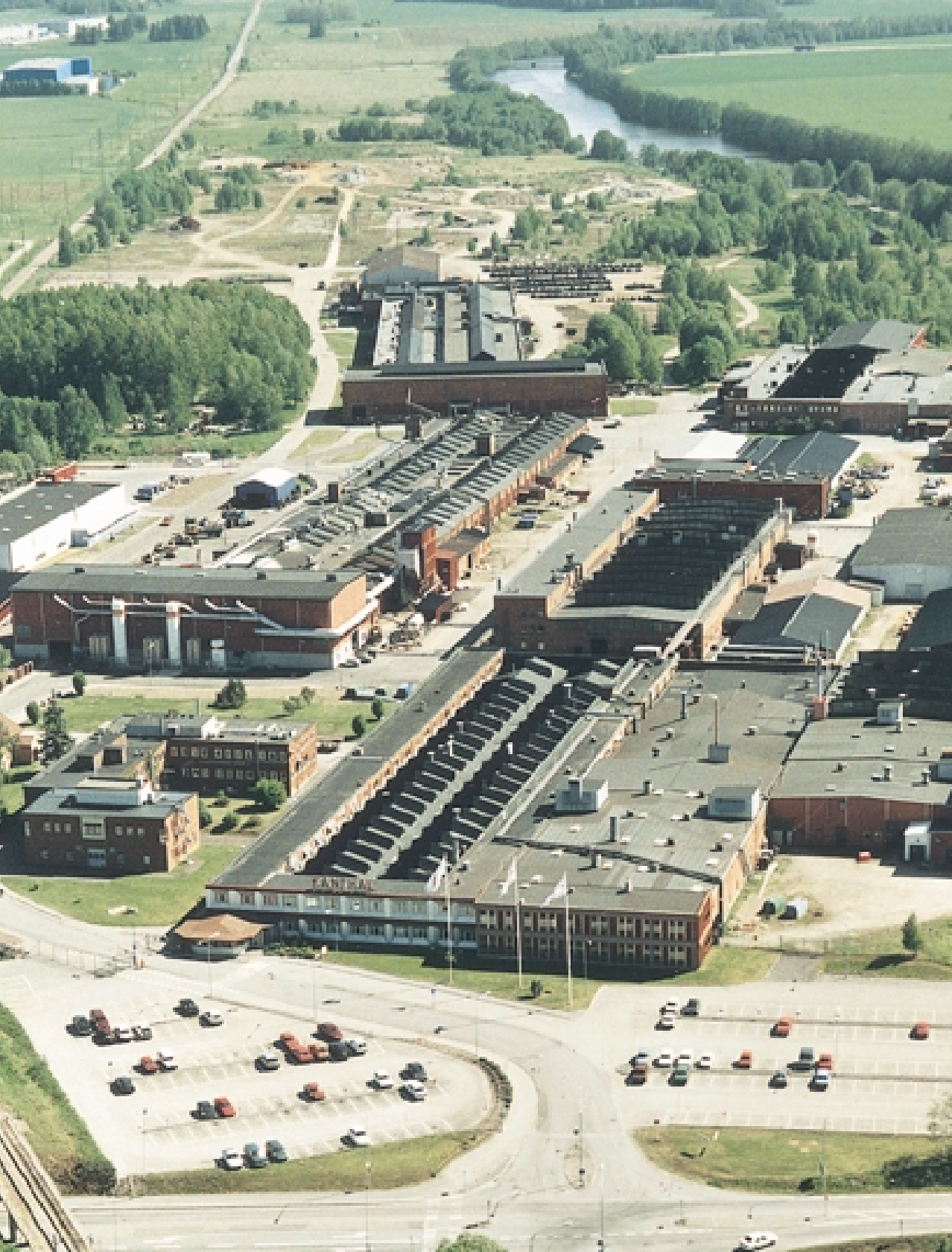
The Kanthal Head Office and main plant in Hallstahammar, Sweden.
